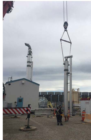
Tower installation on the capture unit.
