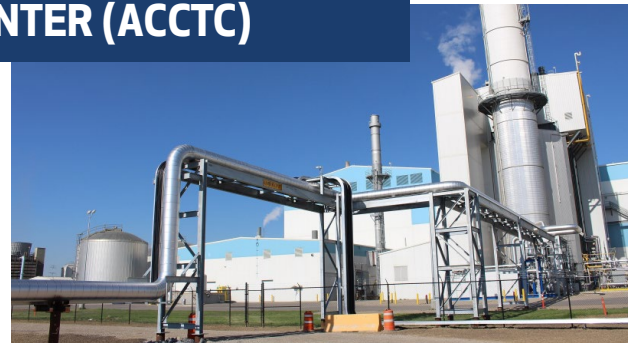
Flue gas delivered from Shepard Energy Centre to ACCTC
