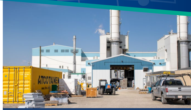
One of ACCTC's six bays occupied by a tenant.
